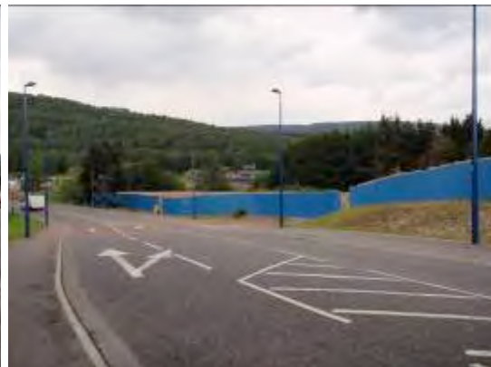
Fig. 2- Link road showing access
